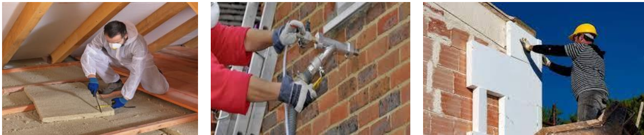
Figure 3: Installation of attic insulation (left), cavity insulation (right), and external wall insulation
